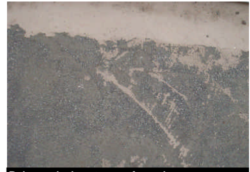
Balcony deck waterproof membrane.
