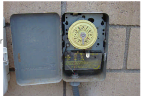
Time clock is lacking pins to set time.
