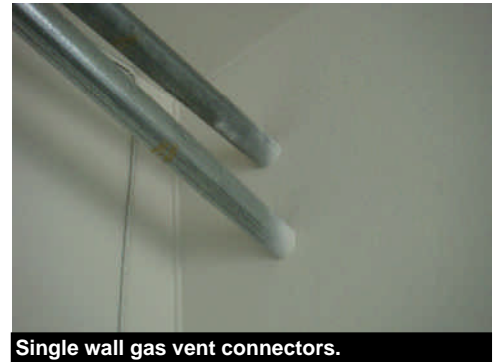
Single wall gas vent connectors.
