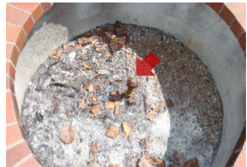
Water came out of the pipe when operating.
