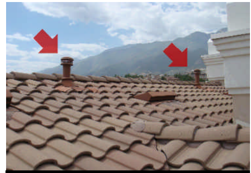
View of the furnace flues at the rear.
