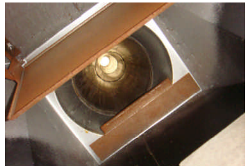
View of the living room flue & damper.
