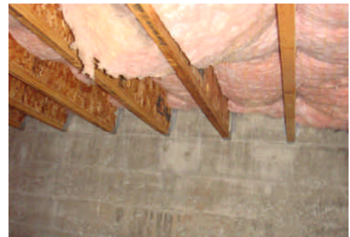
View of the foundation adjacent to planter
