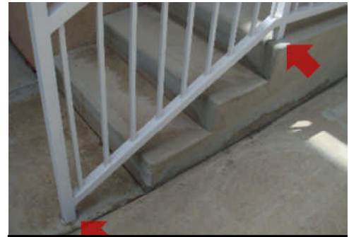
Berm posts and concrete.
