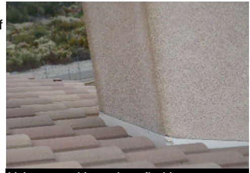
Living room chimney base flashing.
