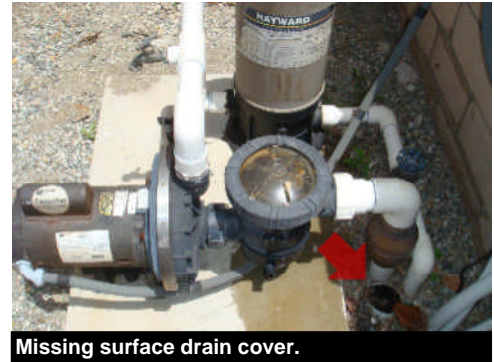
Missing surface drain cover.
