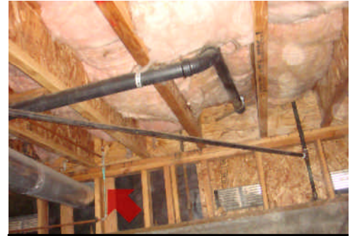
View below the kitchen.
